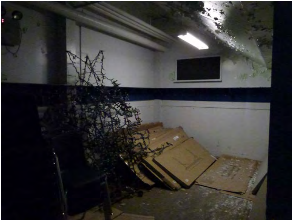
Typical condition of locker/storage rooms.
