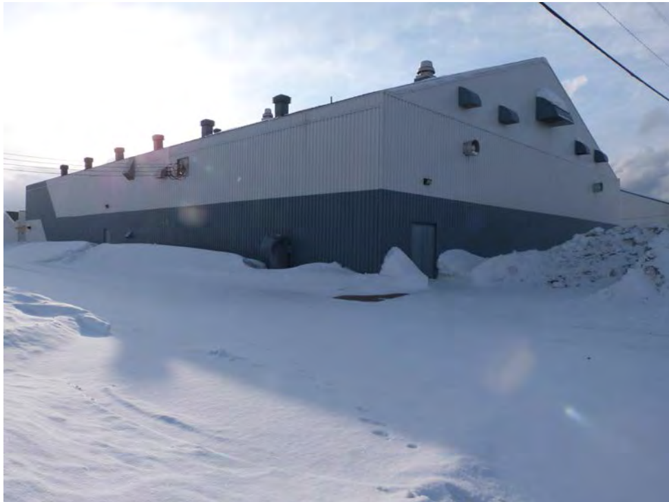
Rear view of training centre.
